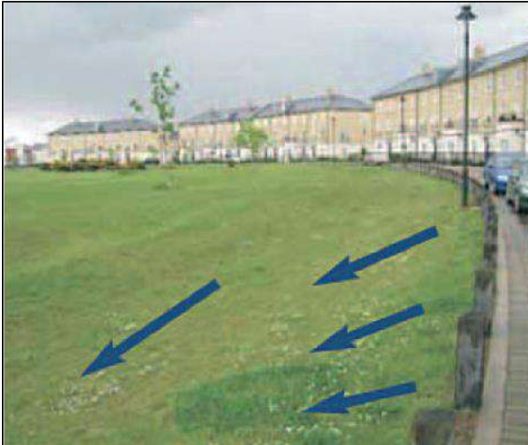
Figure 9: Example of runoff from highway into a basin (Source: taken from Suffolk County Council Local SUDS Design Guide)
